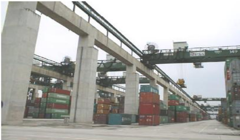
<Figure 3-4> Bridge Cranes Established at PPT
