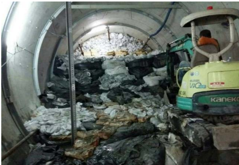
Figure 4. Stacking sandbags to stop water inrush in the tunnel.
