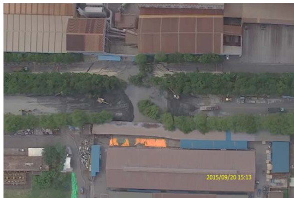
Figure 7. Aerial photo of the hazard-impacted area of the disaster.
